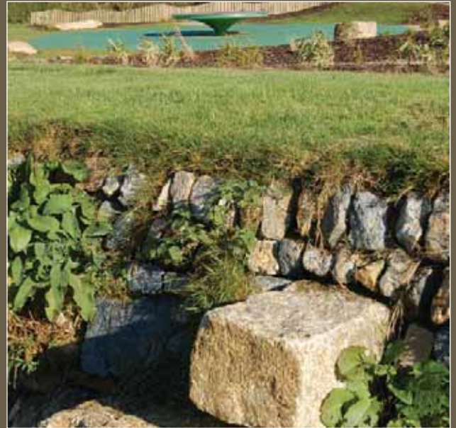
Projecting 'climbable' steps in the dry-stone wall.
